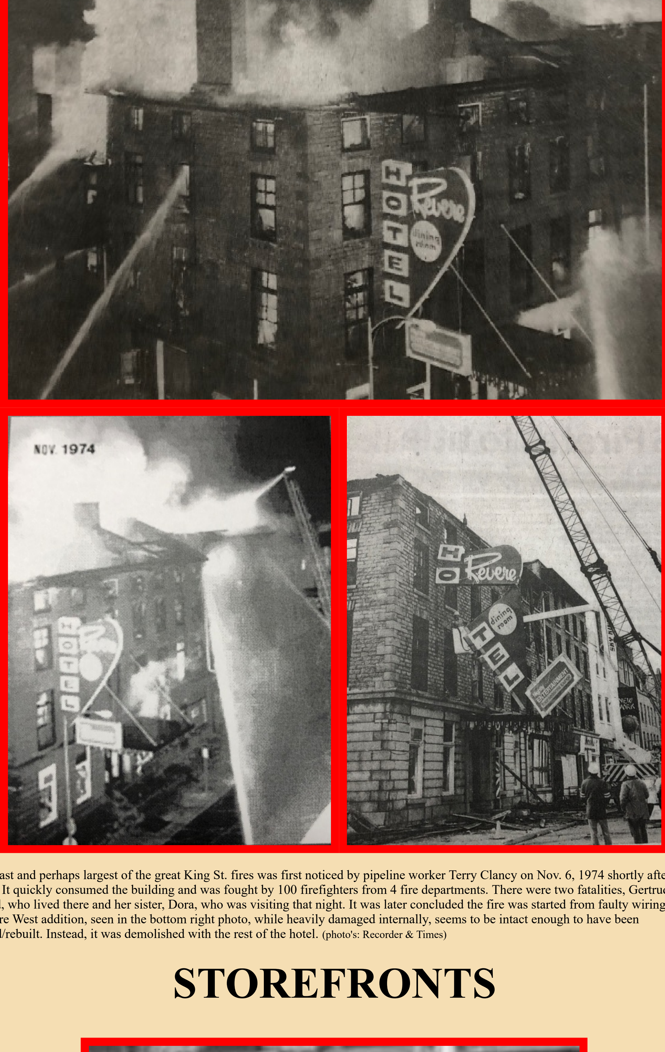
The last and perhaps largest of the great King St. fires was first noticed by pipeline worker Terry Clancy on Nov. 6, 1974 shortly after 9pm. It quickly consumed the building and was fought by 100 firefighters from 4 fire departments. There were two fatalities, Gertrude Steed, who lived there and her sister, Dora, who was visiting that night. It was later concluded the fire was started from faulty wiring. The Revere West addition, seen in the bottom right photo, while heavily damaged internally, seems to be intact enough to have been saved/rebuilt. Instead, it was demolished with the rest of the hotel. (photos: Recorder & Times)
