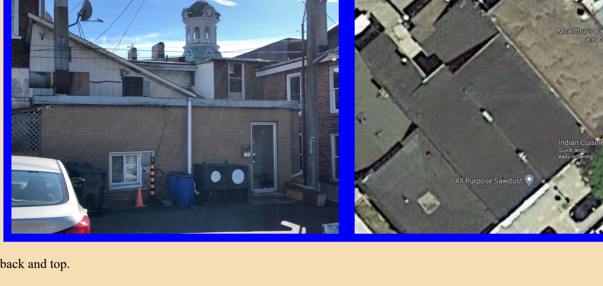
This building from the back and top.
